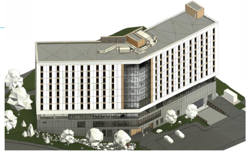
900 Fifth Street ($55.9 million - Phase 2) - 10 storey student residential housing building (VIU)
