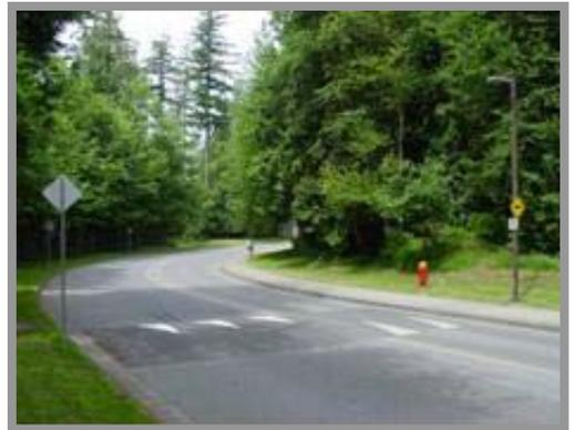
**Disbenefits:** May reduce response times by 1 to 10 seconds per hump. Potential for increased noise due to braking and acceleration. Increases time needed for street sweeping and snow removal. Interferes with pavement overlays. Traffic may be diverted to parallel routes without traffic calming measures. To be used only where other devices are not suitable or sufficient.
