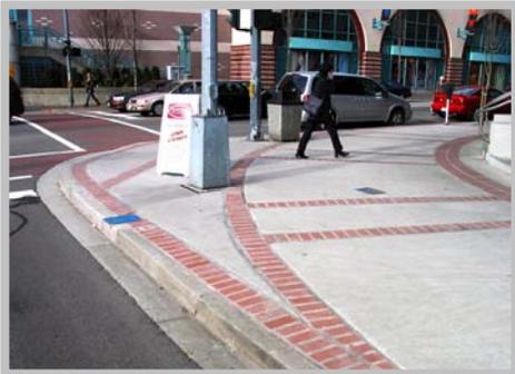
**Disbenefits:** Large vehicles must be considered and curb radius reductions are discouraged on transit routes. There is the potential for rear-end collisions due to right turning vehicles rapidly decelerating.
