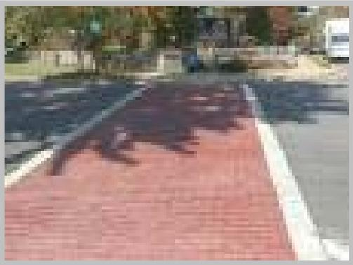
**Disbenefits:** Increases time to street sweep if deep grooves are present. Increases noise levels. When rough or pronounced grooves are parallel to direction of travel, traction and stability problems are created for seniors, the disabled, wheelchairs, bicycles and motorcycles. Can be costly to construct and maintain.
