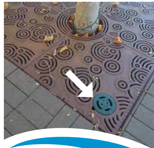
Power and potable water hook-ups are located throughout Spirit Square in removable tree grate covers to facilitate events set-up and reduce the need for stringing power cords across the plaza.
