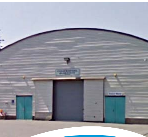
The Centennial Building is a popular covered sport space and is also heavily booked by the Nanaimo Kennel Club and for special events.
