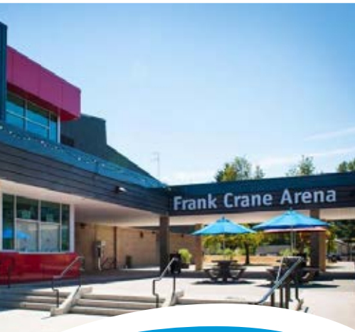
Improvements to Frank Crane Arena were implemented as part of Option 1.
