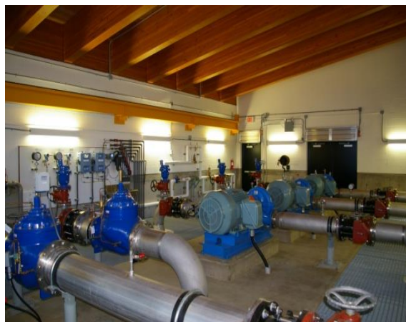
Turbines inside the Energy Recovery Facility
