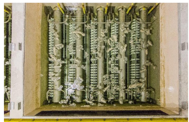
Raw water being filtered in primary membranes
