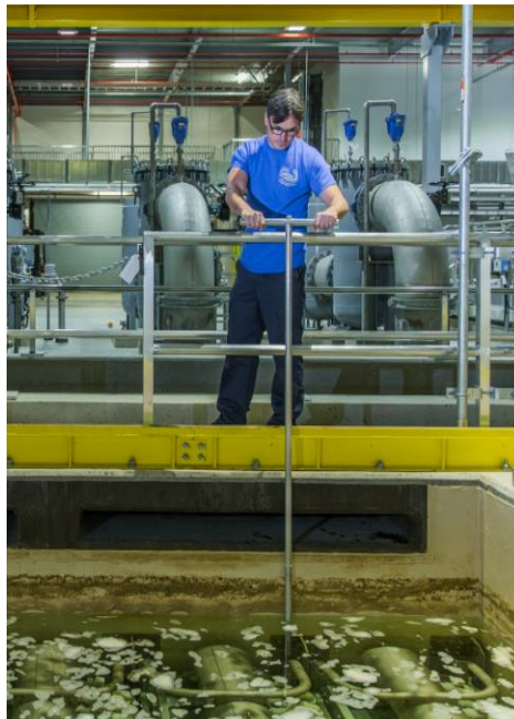
South Fork Water Treatment Plant – primary membranes
