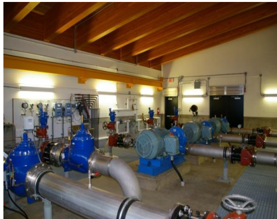
Turbines inside the Energy Recovery Facility
