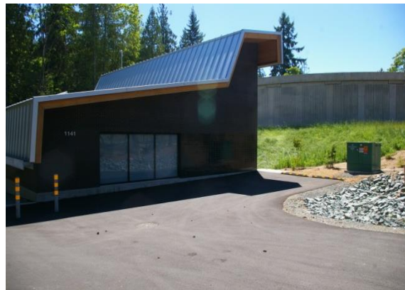
The Energy Recovery Facility and the Reservoir #1 drinking water storage tank (in the background)
