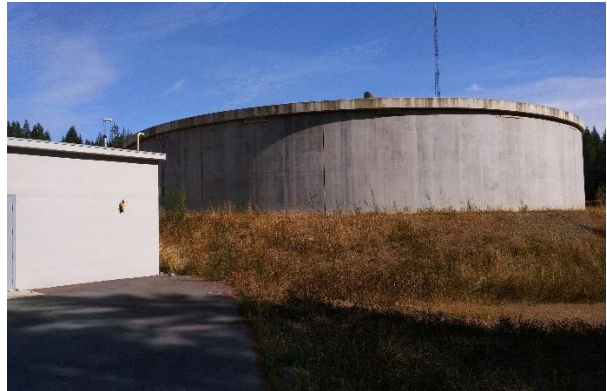
Treated potable water clearwell (storage tank)
