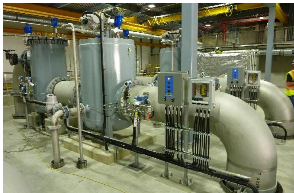
Raw water passes through coarse & fine screens
