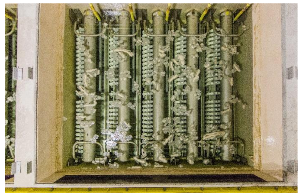
Raw water being filtered in primary membranes
