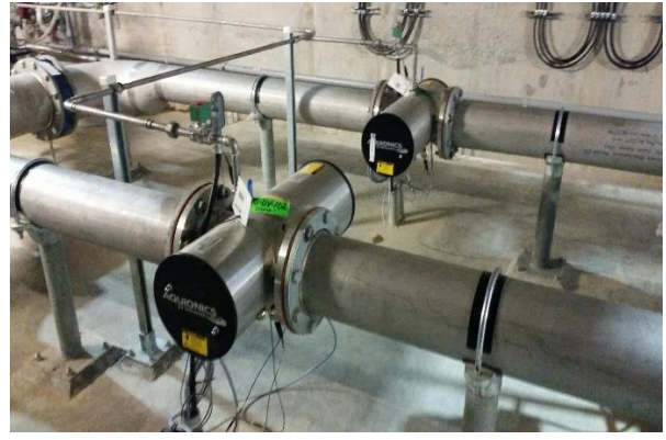
Secondary membranes raw water uv treatment
