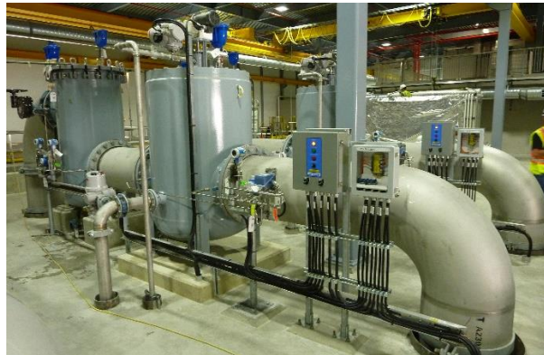
Raw water passes through coarse & fine screens
