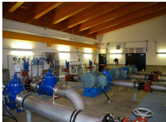
Turbines inside the Energy Recovery Facility
