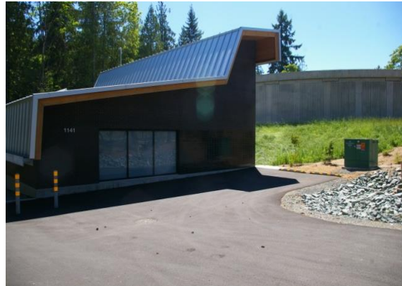
The Energy Recovery Facility and the new Reservoir #1 drinking water storage tank (in the background)
