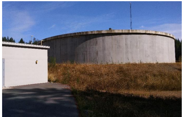
Treated potable water clearwell (storage tank)
