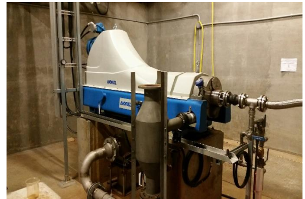
Reject raw water centrifuge
