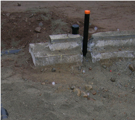
Underslab Plumbing & Radon Piping
