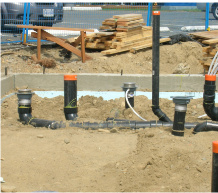
Underslab Plumbing & Radon Piping
