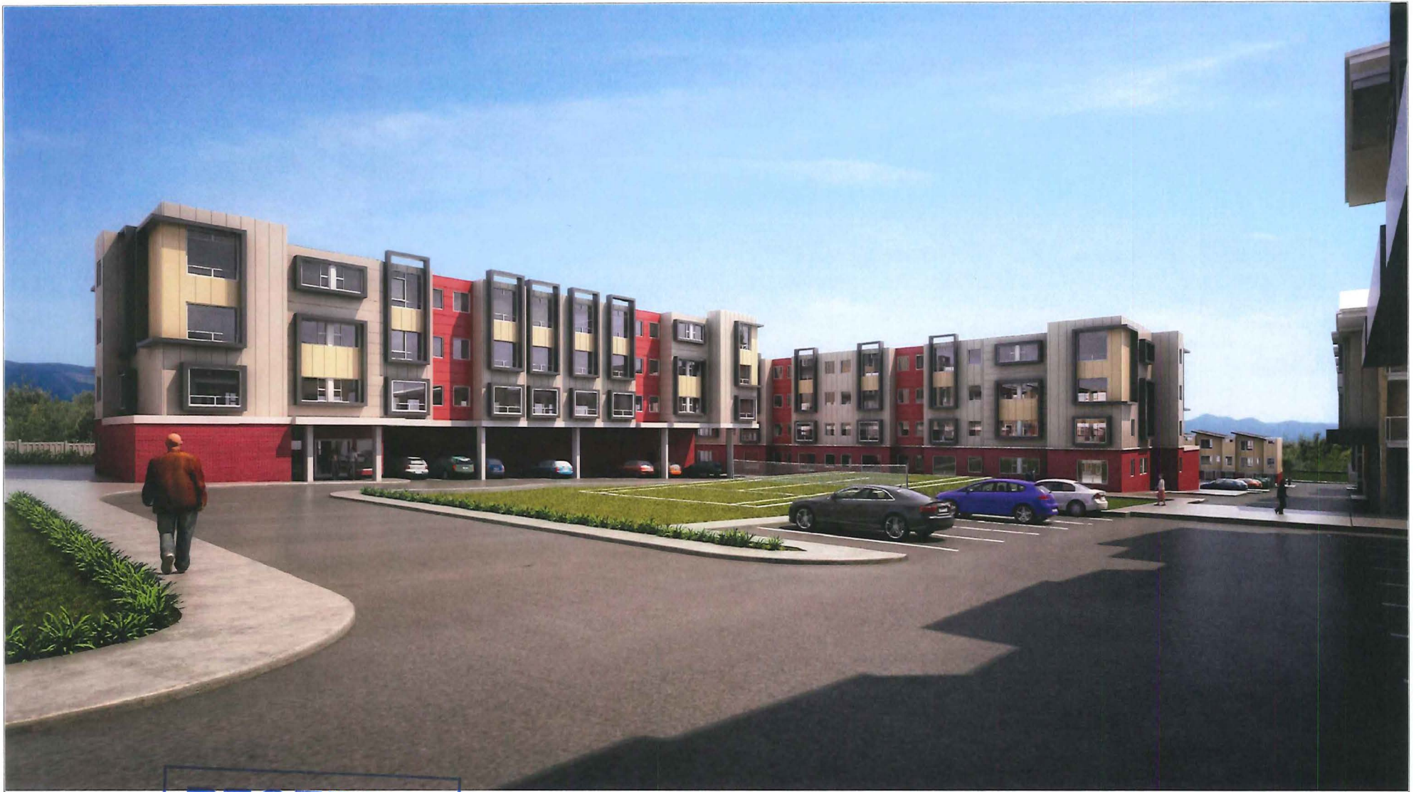
INTERIOR BUILDING VIEW
