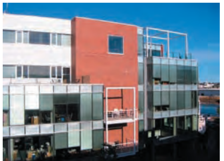
Cladding options include brick, glass, metal, stone and concrete.
