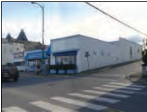
B. SOUTHWEST AT CHAPEL & FRONT
