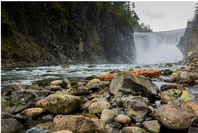
South Fork Reservoir
