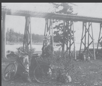
◀ WINNIE GLAHOTMY E&N RAILWAY TRESTLE, LATE 1800'S
