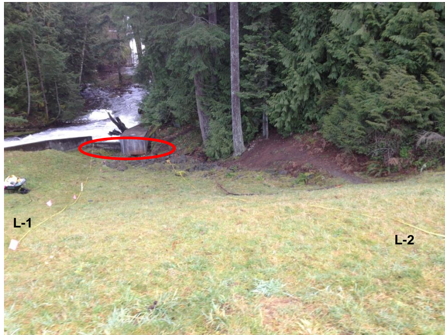
Photograph B-5: Middle Dam—from the crest, looking down the face between lines L-1 and L-2 marked by measuring-tapes. Bedrock outcrop occurs within the red circled area and spans the floor of the spillway.
