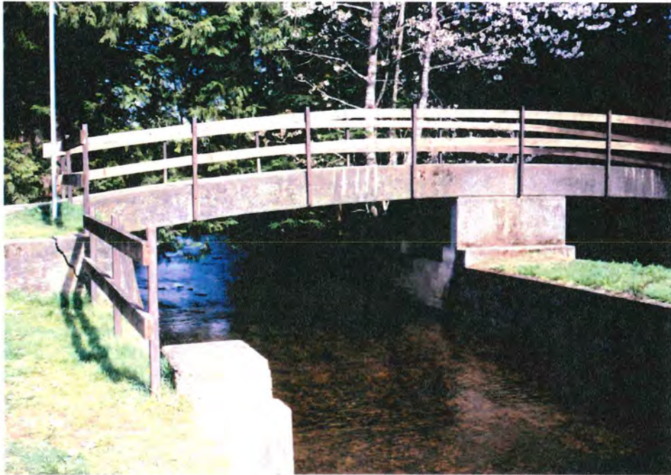
CONCRETE FOOTBRIDGE OVER CONCRETE SPILLWAY
