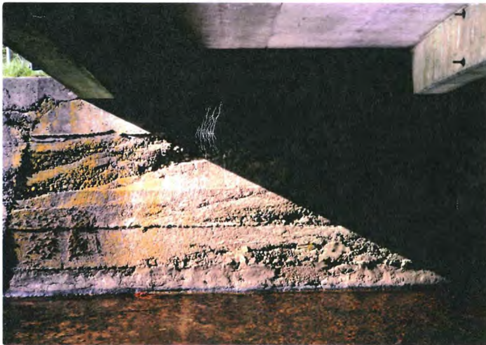
OLD CONCRETE SPALLING AND SEGREGATED BENEATH FOOTBRIDGE AT SPILLWAY
