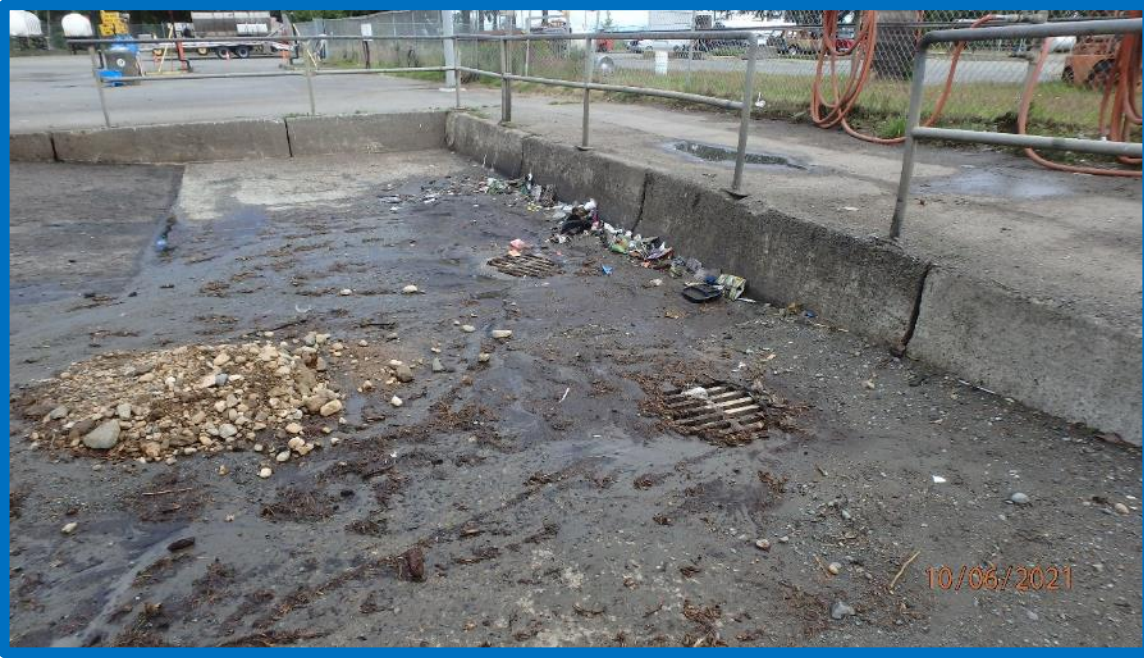
Image 17 Garbage Truck Wash Down Area Drainage
