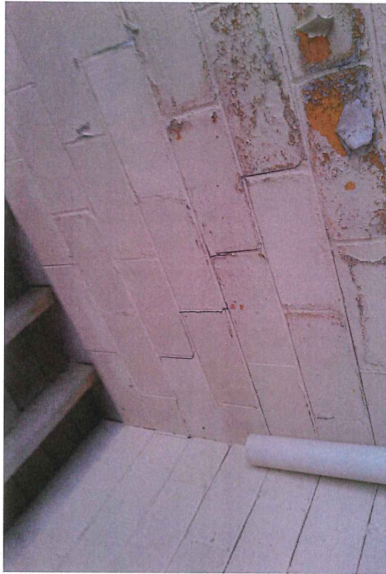
STRESS FRACTURES IN OPEN BAY-- EAST WALL
