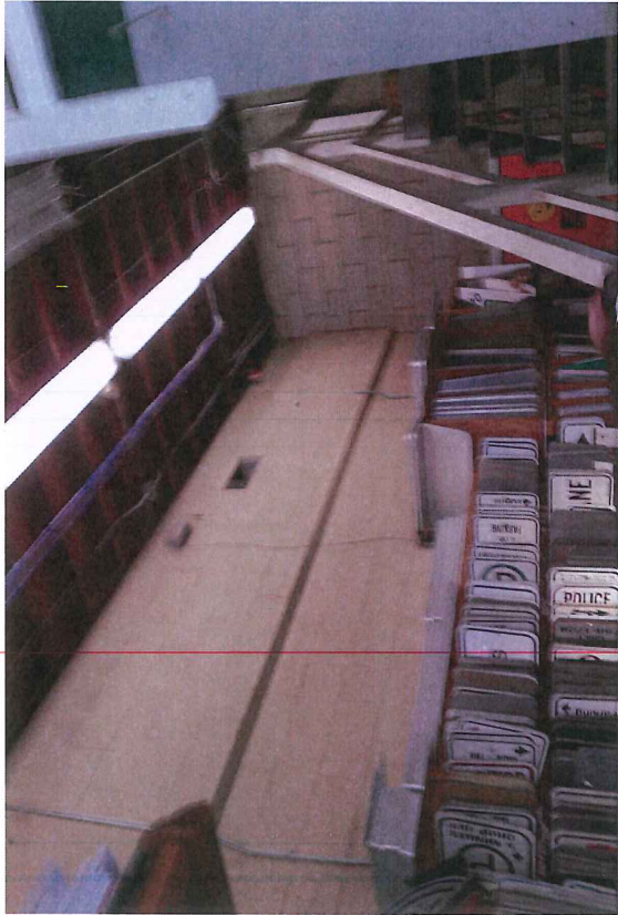
INTERIOR CONCRETE BLOCK PARTITIONS
