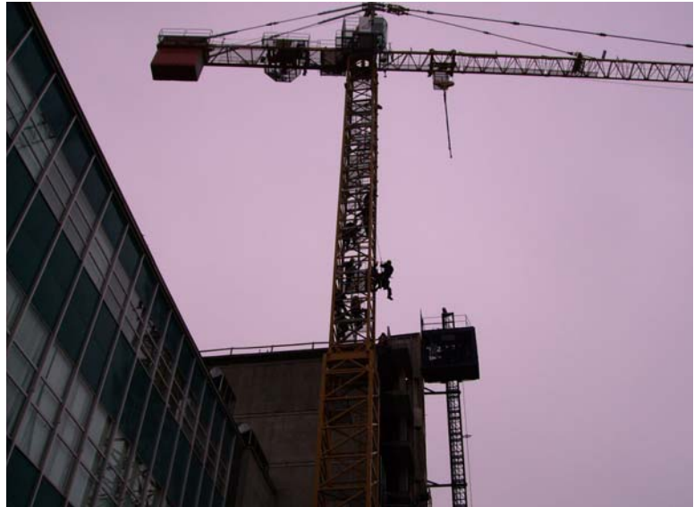
Crane Training Exercise
