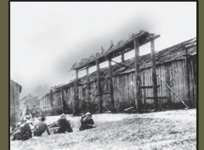
▲ Long House at Departure Bay
