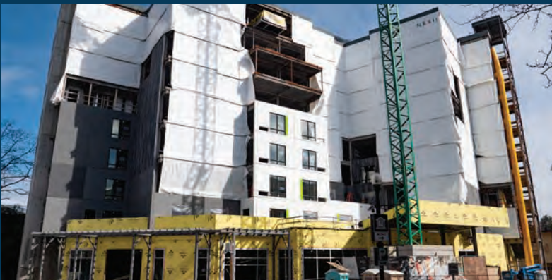
New Marriott Courtyard Hotel under construction
