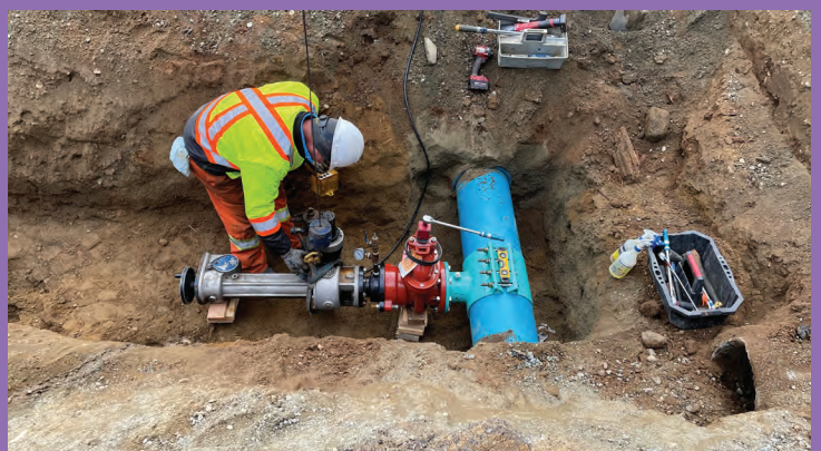
Water main tie-in
