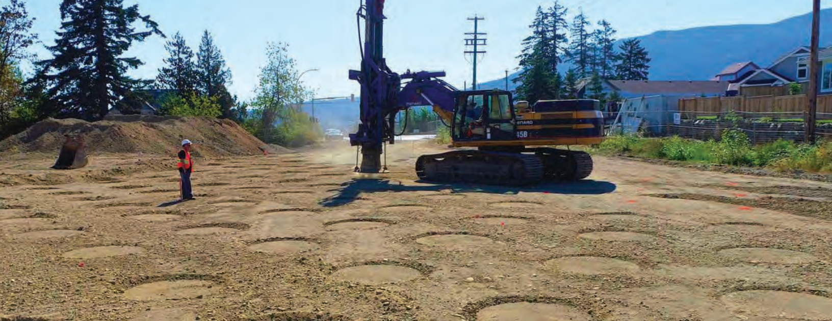
Site prep (rapid impact compaction) for Midtown Gateway project
