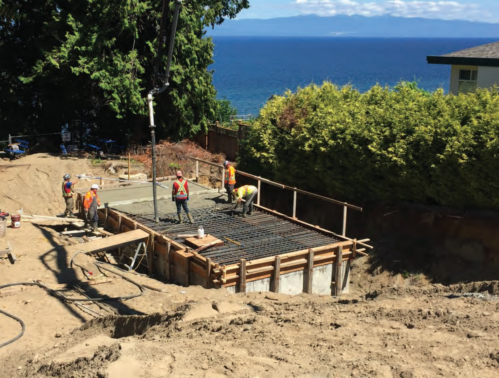
Concrete chamber built for Seabold Drainage project
