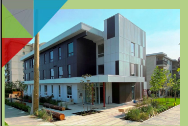
Supportive Housing in Nanaimo
